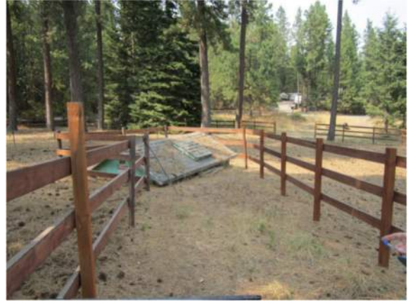
Photo 2: Existing Snowshoe Booster Station
