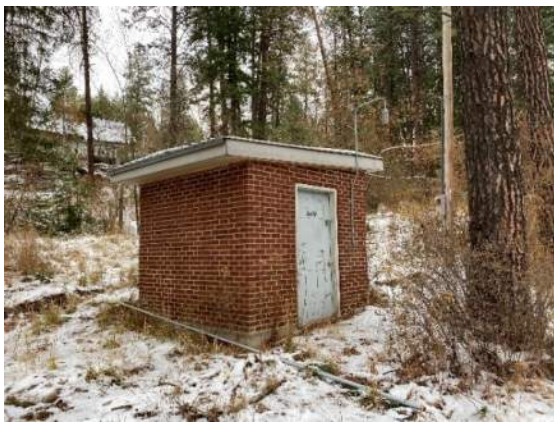
Photo 7: Upper Highland Booster Station
